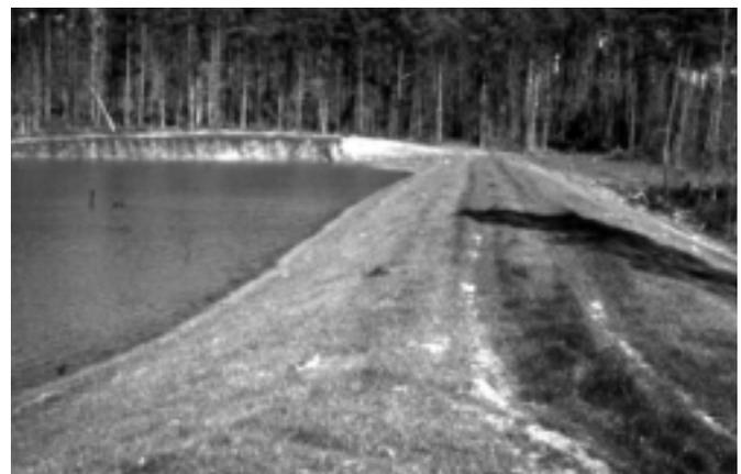
**Figure 15.** Seed new pond embankments to establish vegetative cover and reduce erosion.
