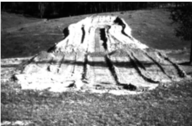
Figure 12. Initial clearing for base of pond dam and cutoff trench
