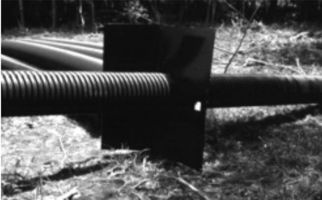
**Figure 7.** Pipe being prepared for installation through dam (barrel pipe) with antiseep collar attached
