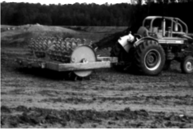
**Figure 14.** Using sheep's foot roller to compact earthfill
